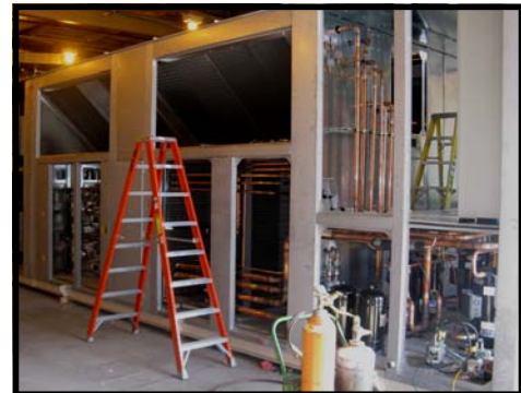
DX-ACCU/Furnace Section
