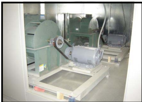
Dual blower and motor configuration
