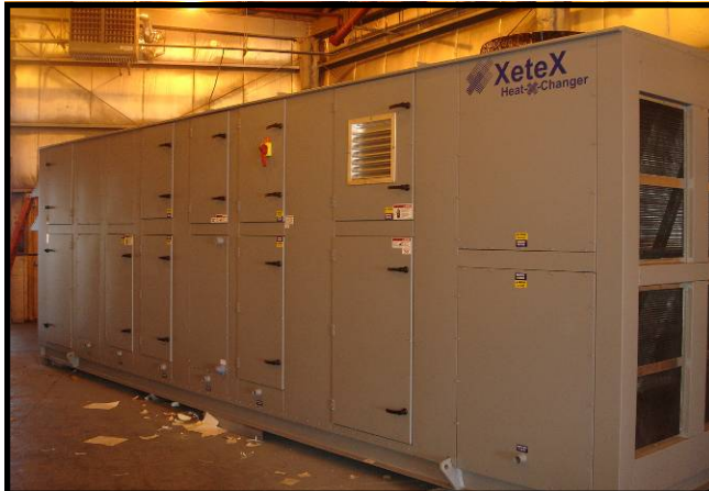
The finished PXHS unit incorporates a full refrigeration circuit.
