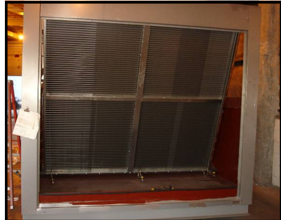
The air cooled condensing section is located on one end of the unit.
