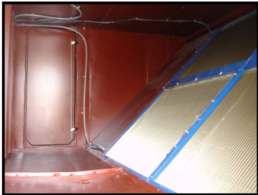
Heresite-Coated Cabinet Interior and Epoxy-Coated Exchanger
