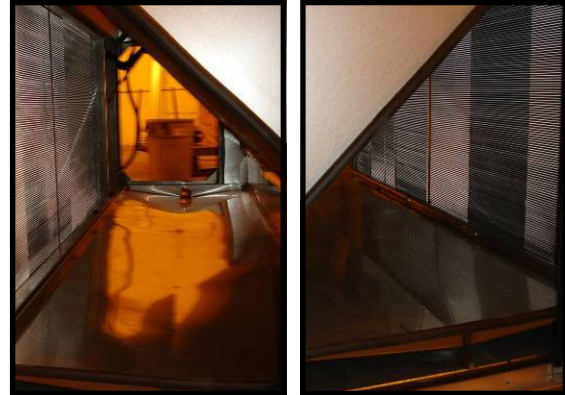
DX Coil for cooling and dehumidification (right), Hot Gas Bypass coil for Reheat (left).
