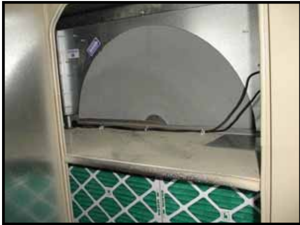
Heat Wheel and Filters
