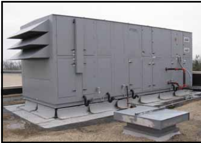
The Finished and Installed PXHS
