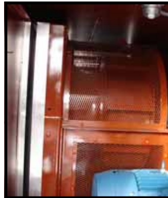
Heresite-Coated Blower and Cage
