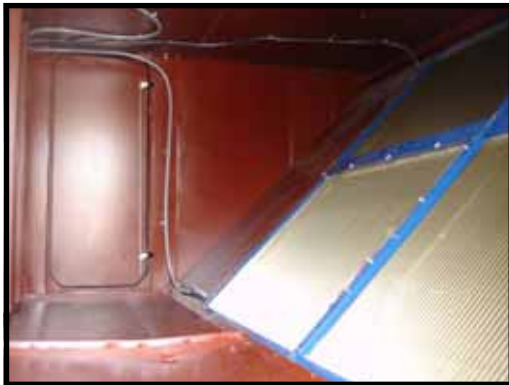
Heresite-Coated Cabinet Interior and Epoxy-Coated Exchanger
